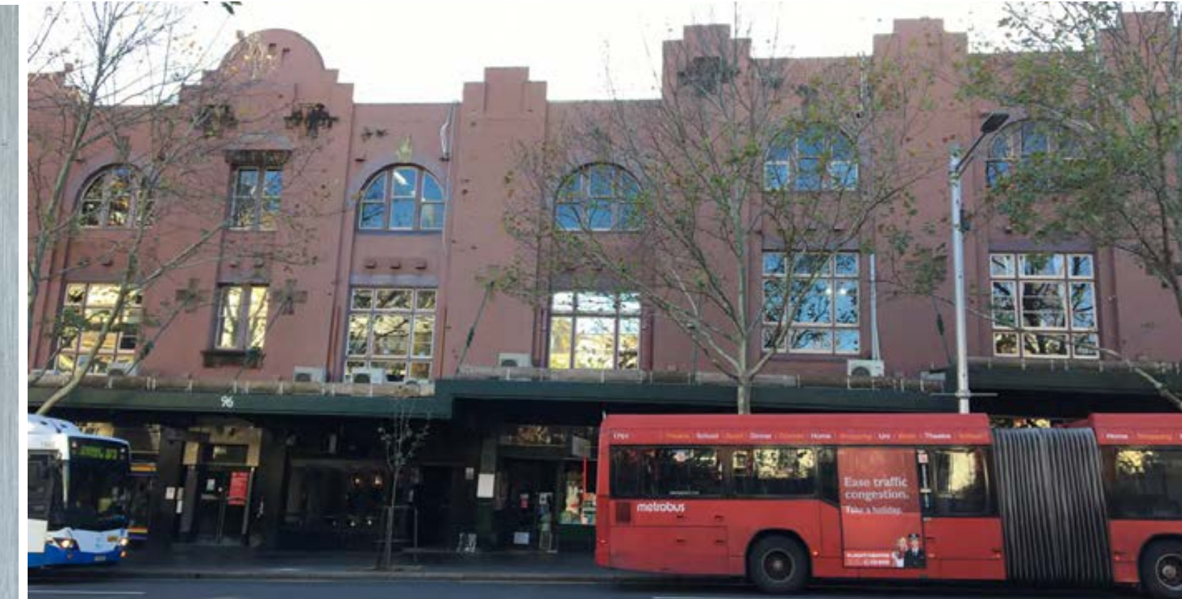
/Existing materiality reference: brickwork to be stripped
